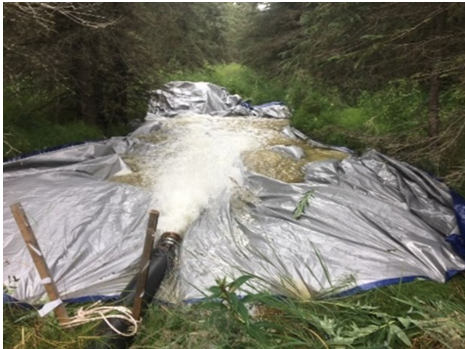
SOP9.3. Pumping water from a pond to drain it
