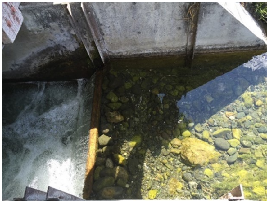
SOP9.1. Water control structure with boards that can be removed to reduce water level
