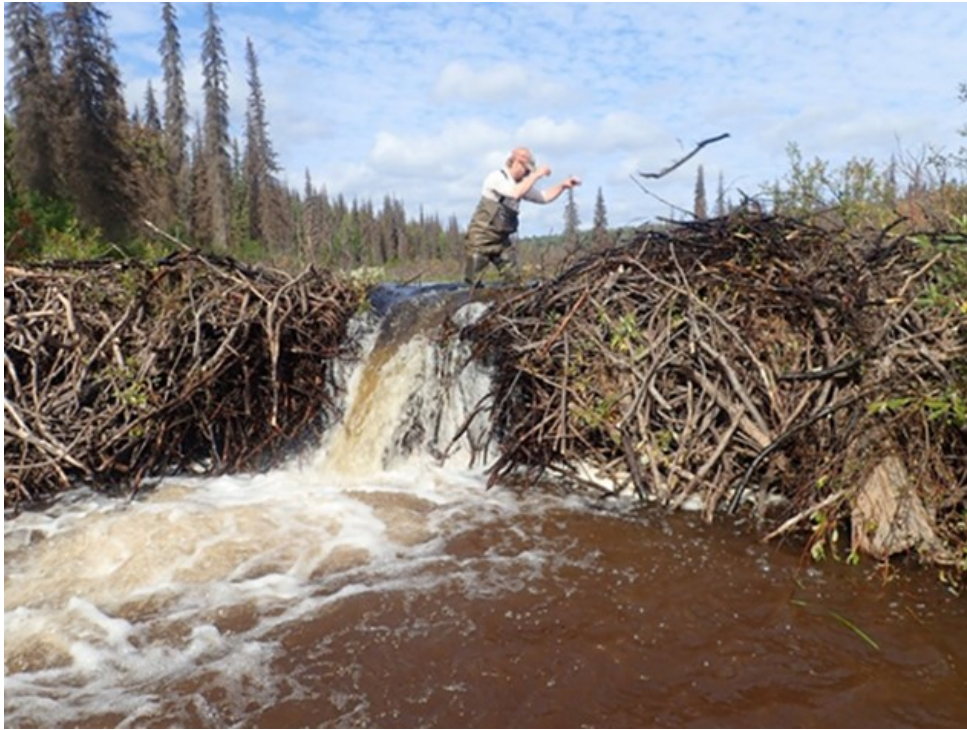
SOP9.2 Notching a beaver dam to reduce water levels
